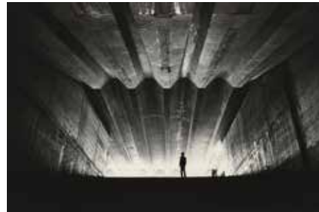
133. David Moore (Aust., 1927-2003). Sydney Opera House, Entrance Under Construction , 1962. Vintage silver gelatin photograph, titled, dated and signed in pencil verso, 19 x 29.5cm. Pinholes, minor missing portions to upper and lower right corners.
