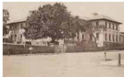
26. Survey Offices [Sydney] , 1871. Albumen paper photograph, numbered "278" in negative centre right, titled and annotated "in 1871" in pencil verso, 17.7 x 27.2cm. Slight foxing overall, surface loss, chips, repaired tears and minor creases to edges.
