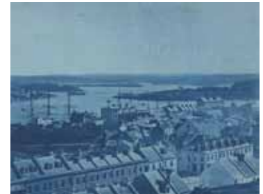
15. [The Rocks, Sydney] , c1880. Cyanotype, 22.1 x 28.3cm. Repaired tear to image upper centre, slight stain to upper left corner, paper remnants verso.
