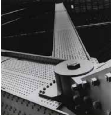
132. David Moore (Aust., 1927-2003). Bridge Structure, Sydney, 1947 . Vintage silver gelatin photograph, titled, dated and signed in pencil, alternate title with date in ink verso, 20 x 19.2cm. Minor scuffs to image, dents and chip to edges of image. $7,700 Alternate title reads "Harbour Bridge Detail."
