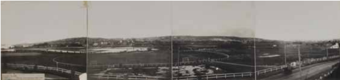
111. Herbert Shaw (Aust., active c1920s). Woollahra Park During Construction [Rose Bay, NSW] , 1929. Silver gelatin photographs, four-panel panorama, title and date typed on label affixed to image lower left, photographer's stamp verso, 15.2 x 77.5cm. Slight soiling, creases and missing portions to edges of image.
