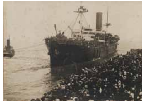
34. [HMAT] Nestor Leaving Port Melbourne Pier , 1916. Silver gelatin photograph, title with date "2.10.16" in ink on label and illegible studio line in letterpress on backing below image, 16.5 x 20.8cm. Tear and surface loss to lower portion, stain to lower centre, slight dents and foxing overall. Laid down on original backing.
